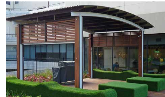
Customised landmark structure note the steel posts faced with timber and prominent steel bolts, create a durable structure with a domestic aesthetic
